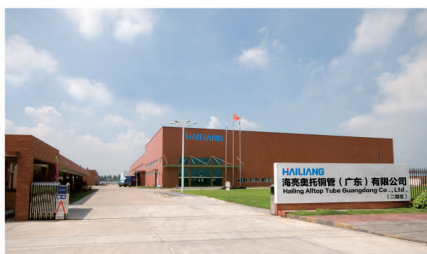
Hailiang Alltop Tube Guangdong Co., Ltd (Plant 2)
