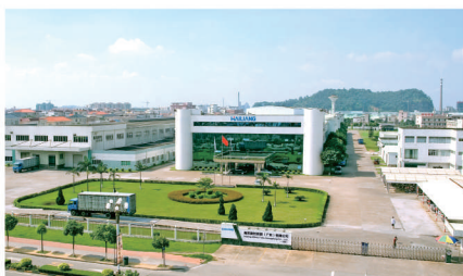
Hailiang Alltop Tube Guangdong Co., Ltd (Plant 1)
